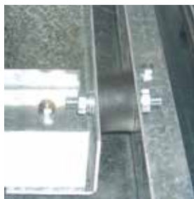
Anti-vibration mounts To reduce vibration and noise transmissions to the installation.
